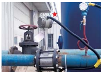
Vortex flowmeter in oxygen measurement
