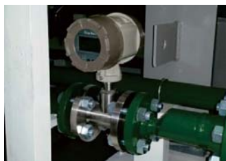
Liquid turbine flowmeter in water supply plant
