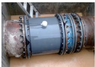
Magnetic flowmeter in under well field
