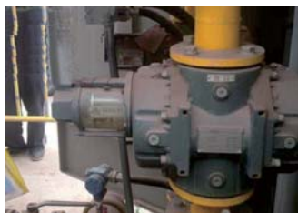
Gas roots flowmeter in gas mixture field
